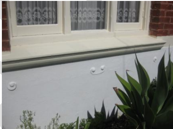
Raise motifs at protruding front room
