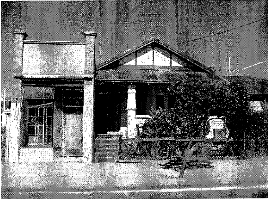
Eastern elevation shop front and attached dwelling
