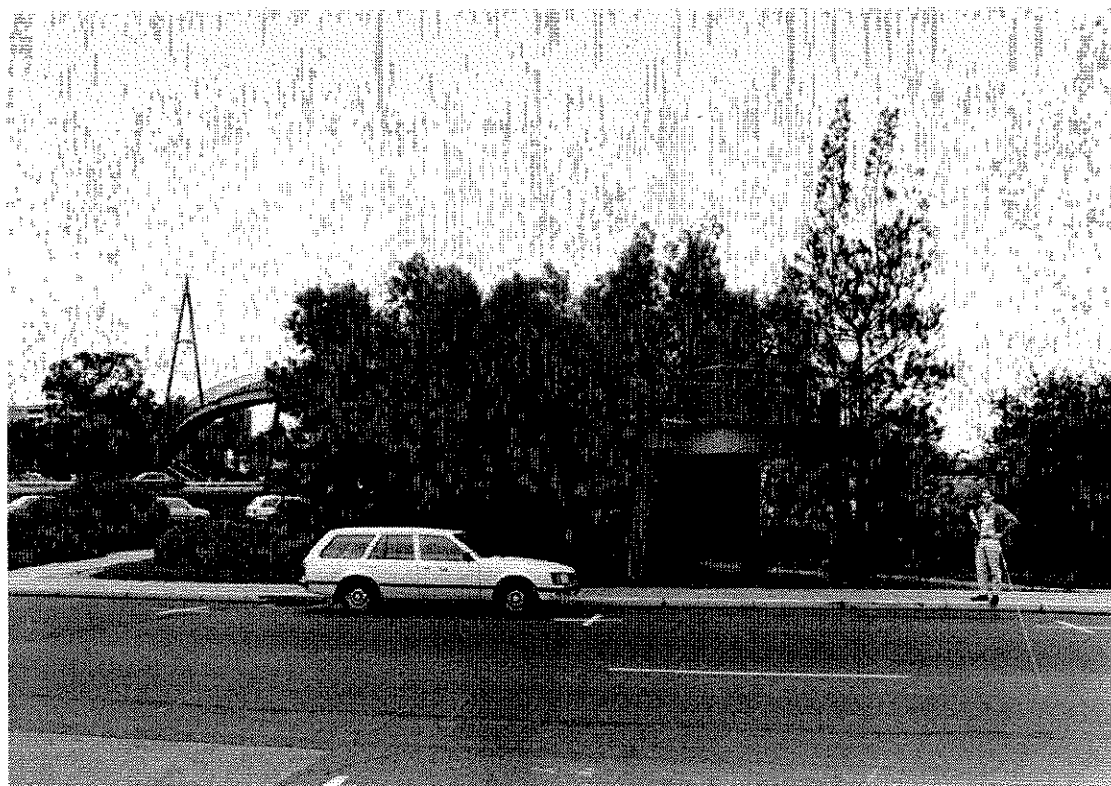
Photo 7: Oxford Street, Leederville, pre 1987.
