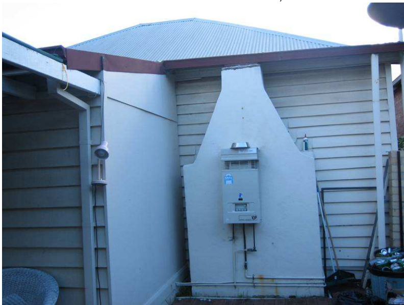
Rear elevation of No. 136 East Parade, East Perth
