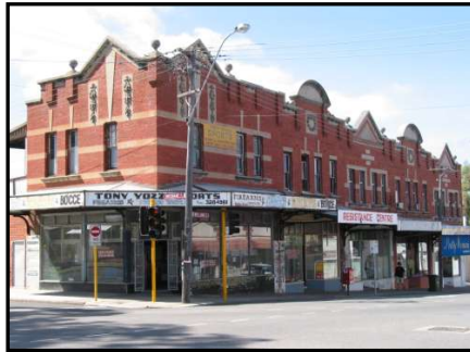
Shop/Houses at Nos. 452 – 460 William Street, Perth
