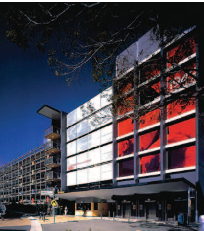
Innovative and attractive screening over public car parks.
