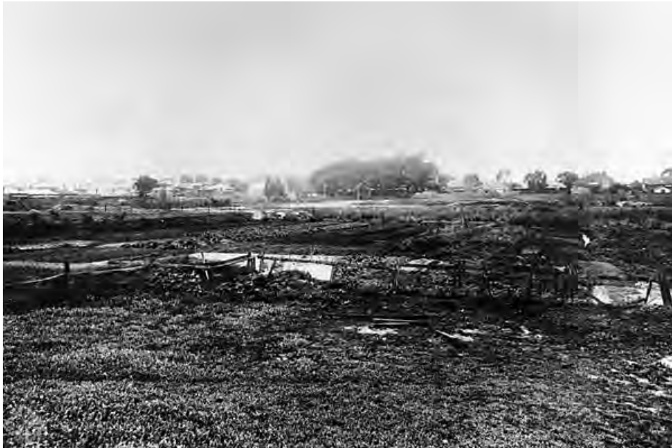
Commencement of works, 1926. Courtesy City of Vincent Local History Collection, Acc No PH00397, image 103794
