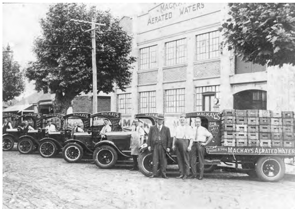
Mackays n.d. Courtesy Mackays Aerated Waters Factory (fmr) Conservation Plan, Palassis Architects, December 2002.
