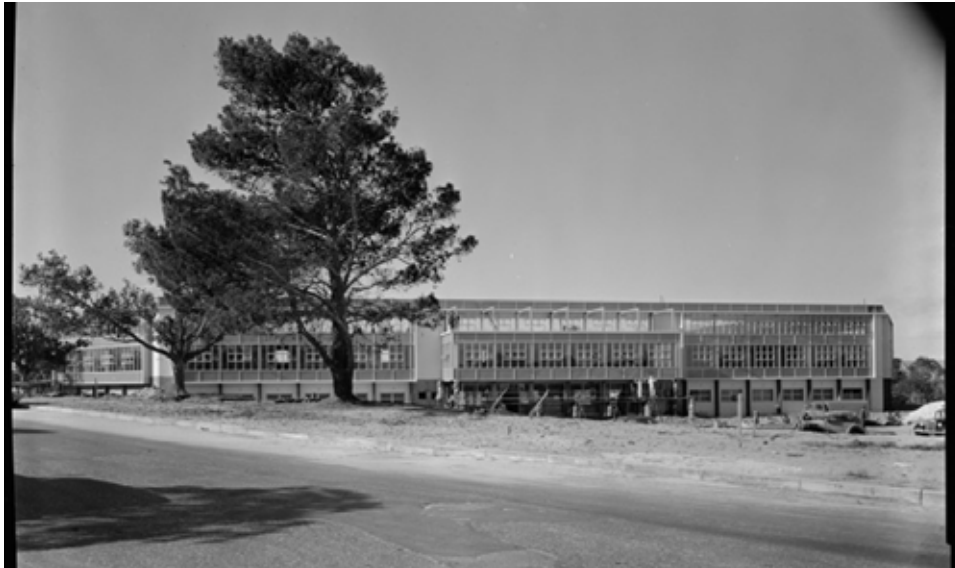
Construction of Beatty Park, 1962. Courtesy SLWA image b3708090_3.
