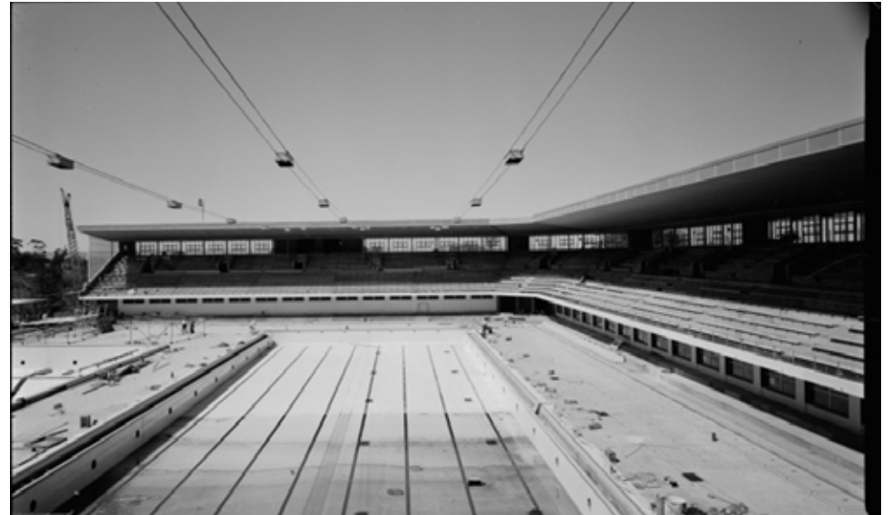
Construction of Beatty Park, 1962. Courtesy SLWA image b3708090_2.
