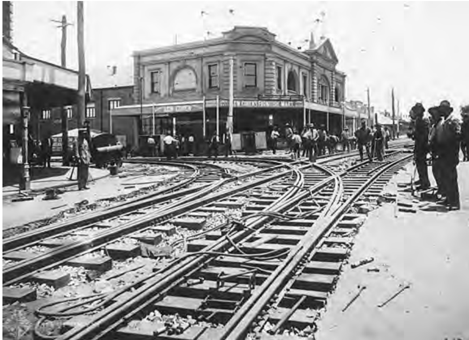
Tramway construction 1931 corner Walcott and Beaufort Streets. Courtesy SLWA image 1028381.
