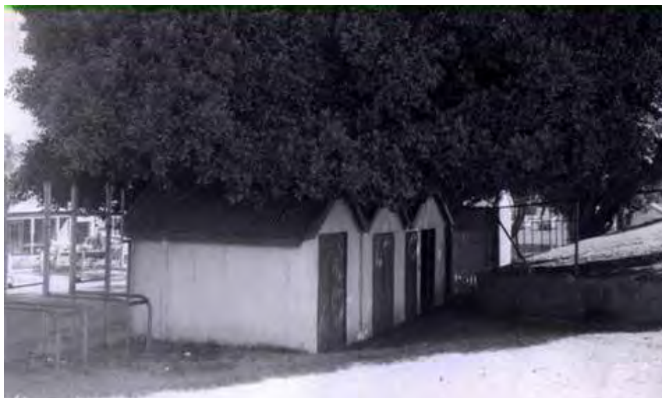
Old Turnstiles, now demolished c1968 Source City of Vincent
