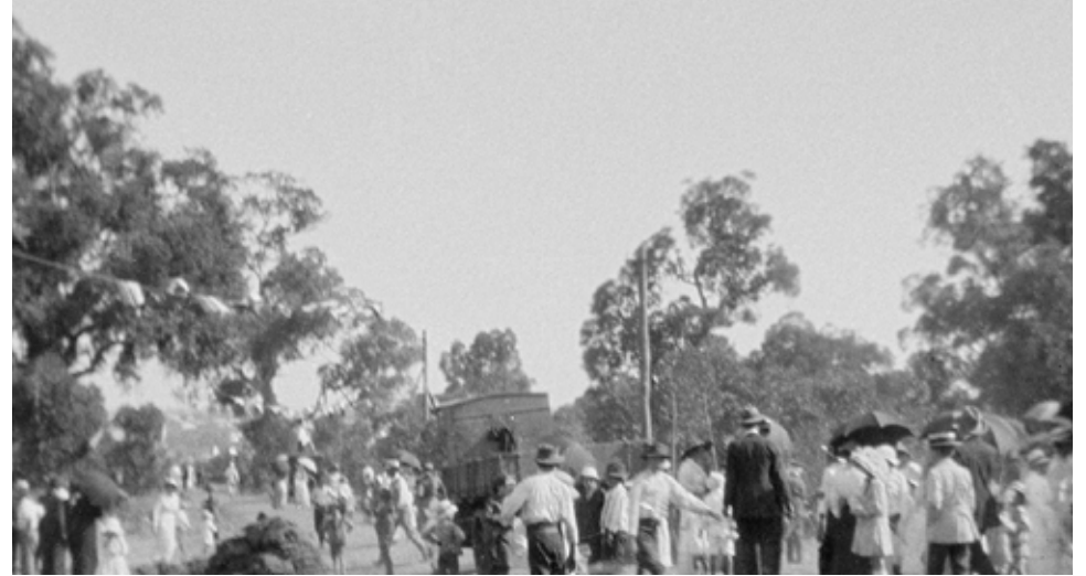
Kalgoorlie Street during the construction of Anzac Cottage, 12 February 1916 City of Vincent
