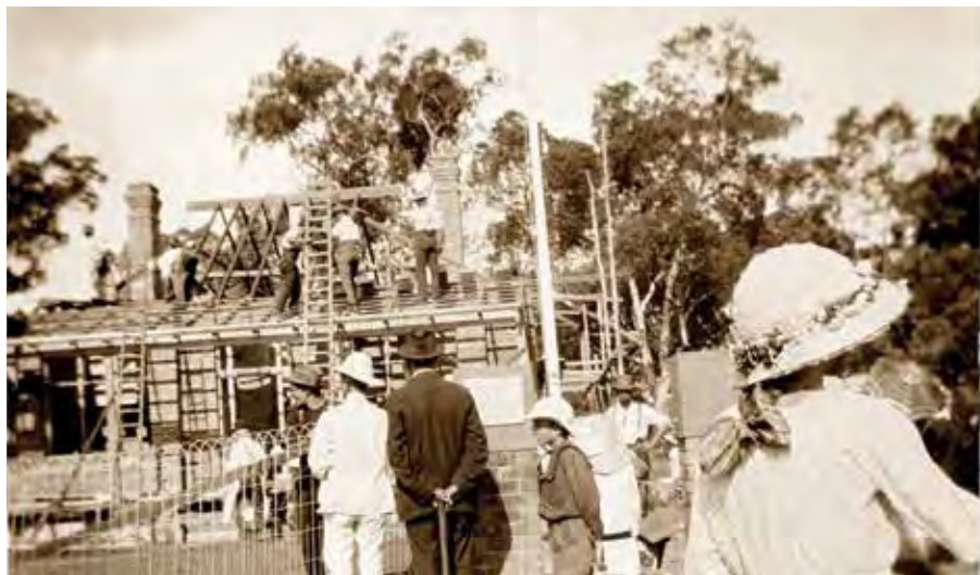
Anzac Cottage construction, 12 February 1916 City of Vincent
