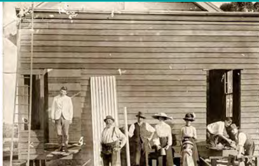
Construction of the Baptist Hall in 1915.
