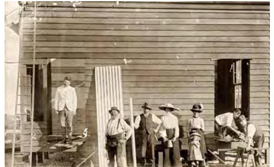
Construction of the Baptist Hall in 1915.
