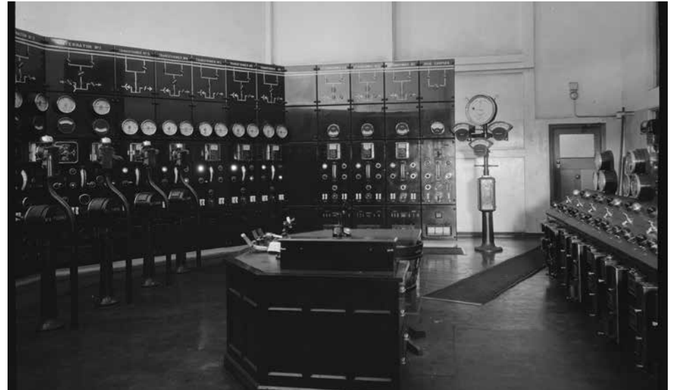
Interior East Perth Power Station 1938. Courtesy SLWA image b2404120_2
