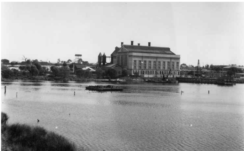
View of East Perth Power Station c1922. Courtesy SLWA image b2194856_2
