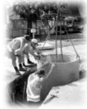
*Facelift for Walcott Street: Engineering Services works crew lower a stormwater drainage manhole liner into position at the intersection of Walcott and William streets, Mt Lawley.*
