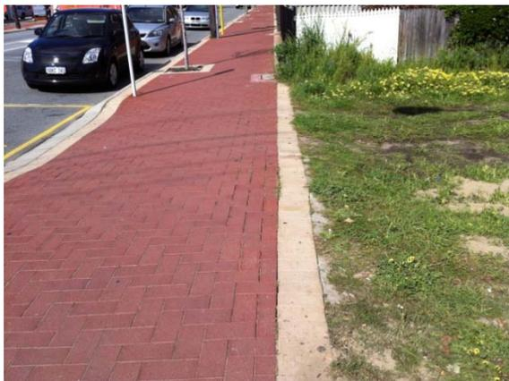
Vehicles are accessing the vacant block from Beaufort Street causing damage to the brick paved footpath.
