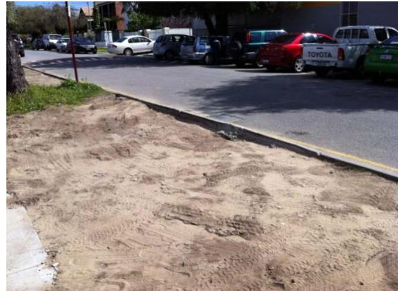
There is a trip hazard (and kerb damage) caused by vehicles continually parking on the verge.
