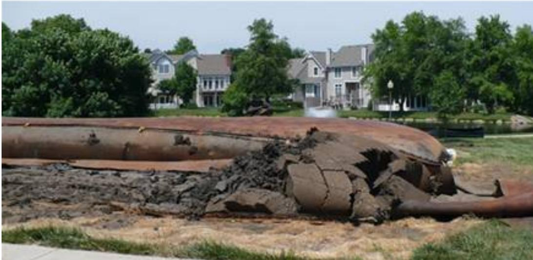
*Envirotubes being cut open to enable the dry material to be removed.*
