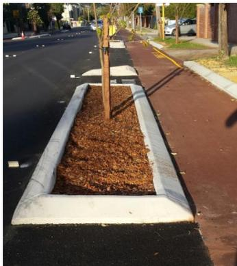
*Figure 2. Sample view of Scarborough Beach Road separated bike lanes*
