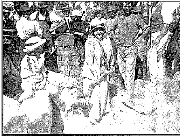
The first trench at Anzac-Mrs C. Roberts, the Soldiers' Queen starting the first trench for foundations
