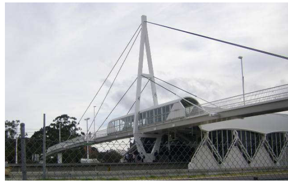
Cable stay bridge structure
