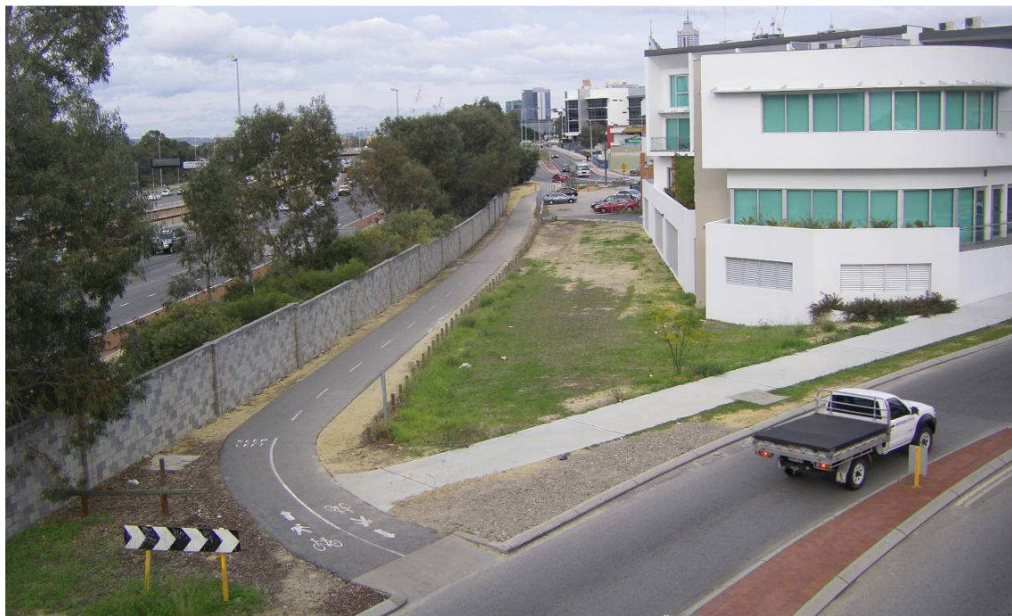
Figure 8 Location of the proposed Leederville Station Bus Interchange Facility (view from the pedestrian bridge)
