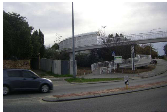
West Leederville (Southport Street) pedestrian bridge connection
