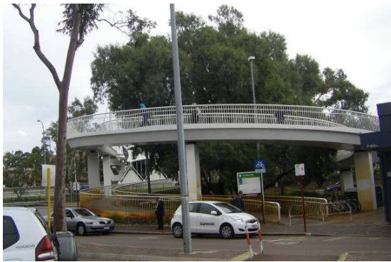
Leederville (Oxford Street) pedestrian bridge connection
