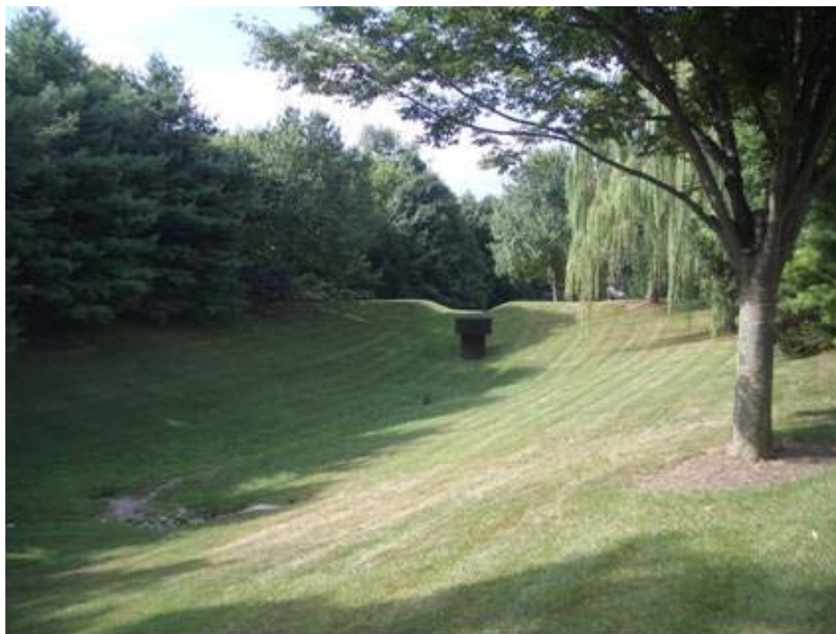
Photo B: Example of a grassed retention basin
