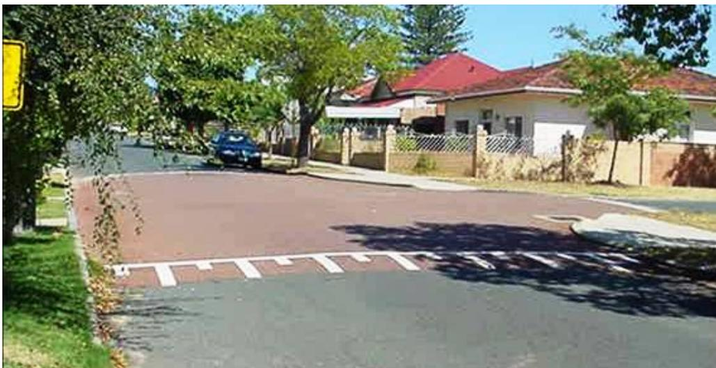
The group finally contended that the installation of a raised plateau at the intersection of Federation and Purslowe Streets (refer example above), would provide a suitable traffic measure to slow vehicle speeds by providing a vertical displacement, together with a visual change at this location.
