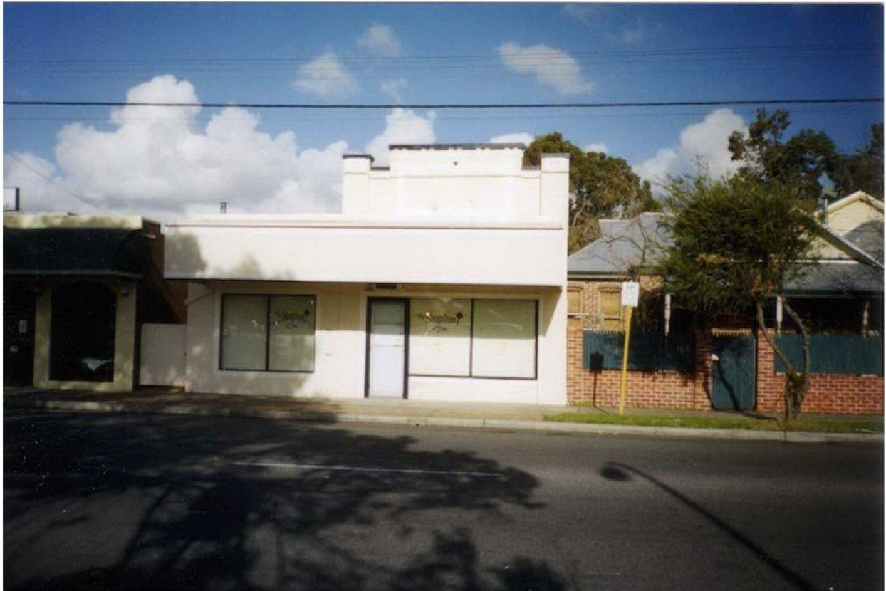
Figure 1: 'The Shopfront' located at 170 Whatley Crescent, Maylands
