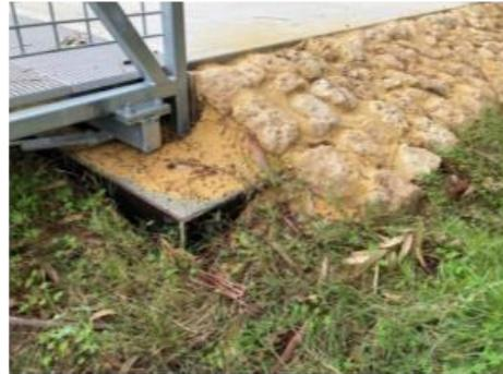
Plate 8 Path erosion protection
