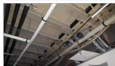
Where partition walls are taken up to underside of suspended ceiling only, the separation performance is less dependent upon the partition and more dependent upon the transmission via ceiling space. Using lightweight mineral fibre ceiling tile on tegular grid, with insulation in the void over, partitions in this arrangement typically achieve Rw 35dB only, which renders loud speech audible/intelligible in adjacent space.
