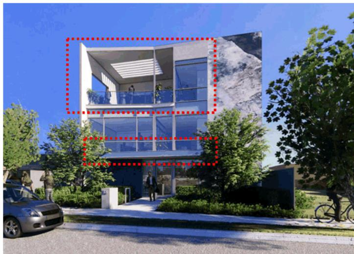
Figure 2.4 - Proposed shading devices
