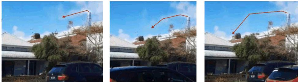
Figure 14: Sequence #2 – plume pushed down by downwash effect
