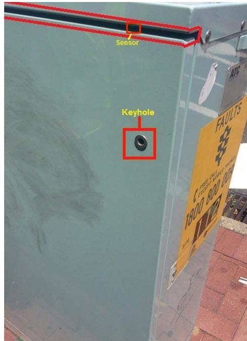
Special care must be taken when painting around the sensor (marked in red).
