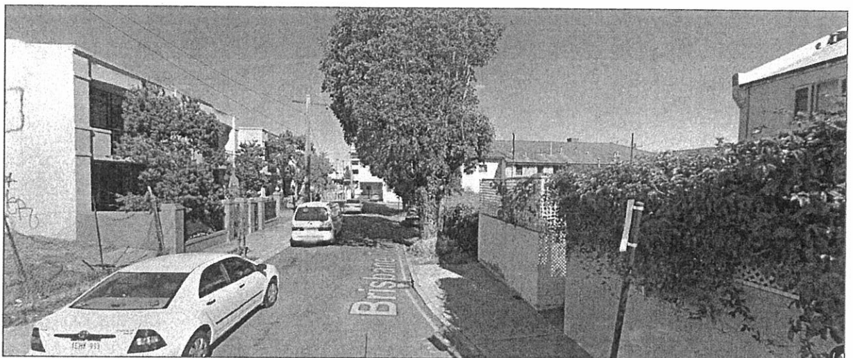
Figure 2 – Existing rear solid street fence of adjoining property – 64A Robinson Ave.
