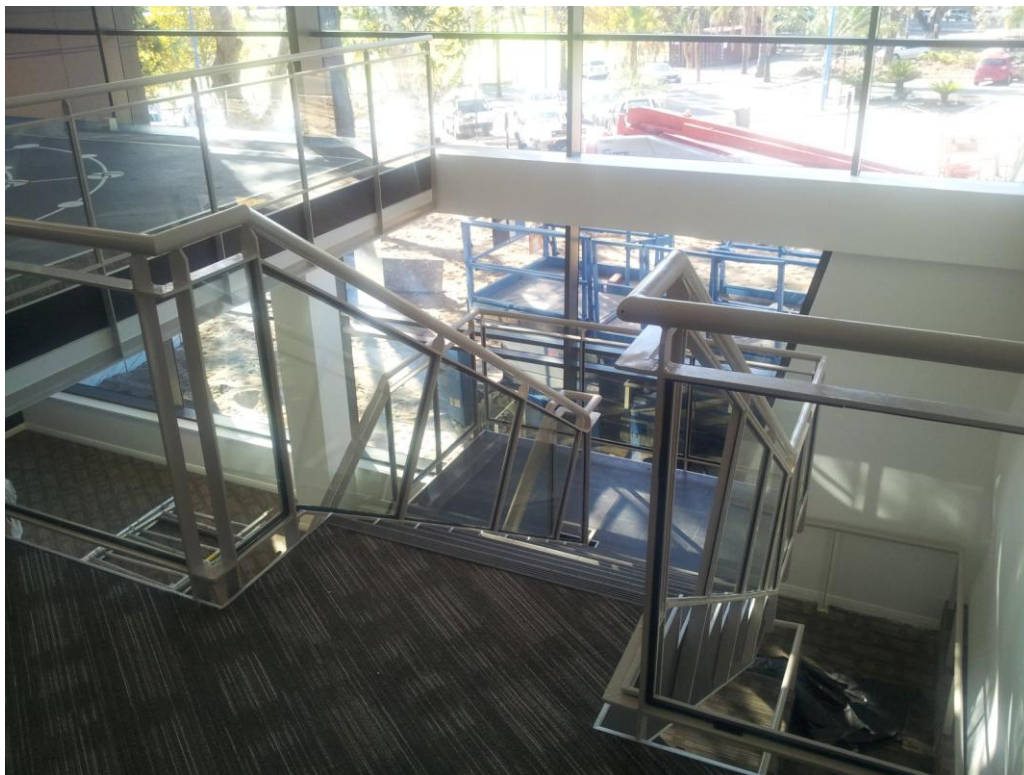
Staircase leading to Gymnasium Entry
