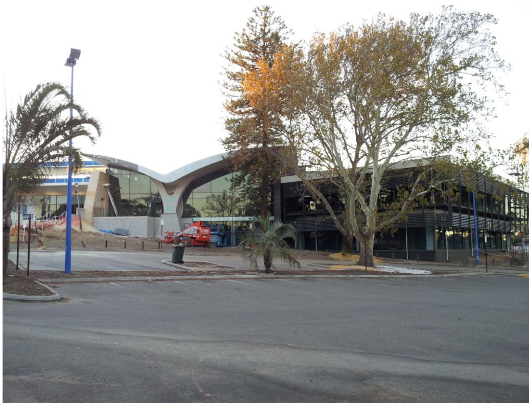
Car Park Works
