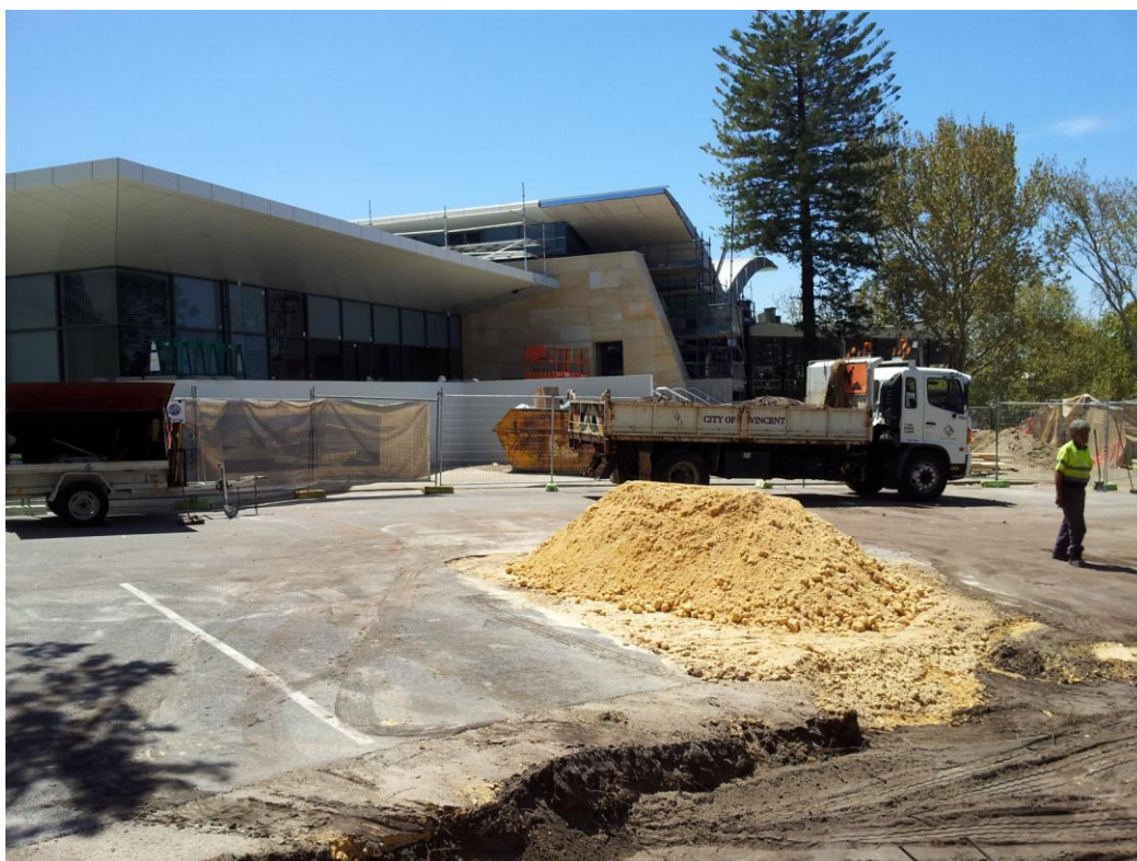
Commencement of Car Park works
