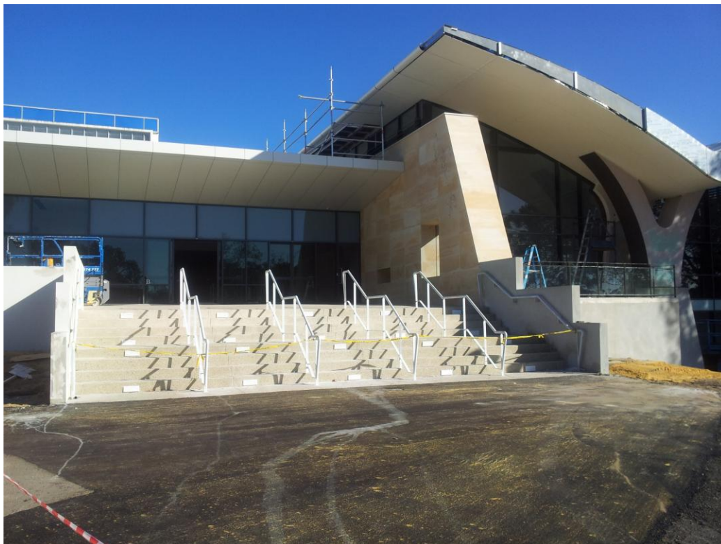
Car Park Works and Front Entry
