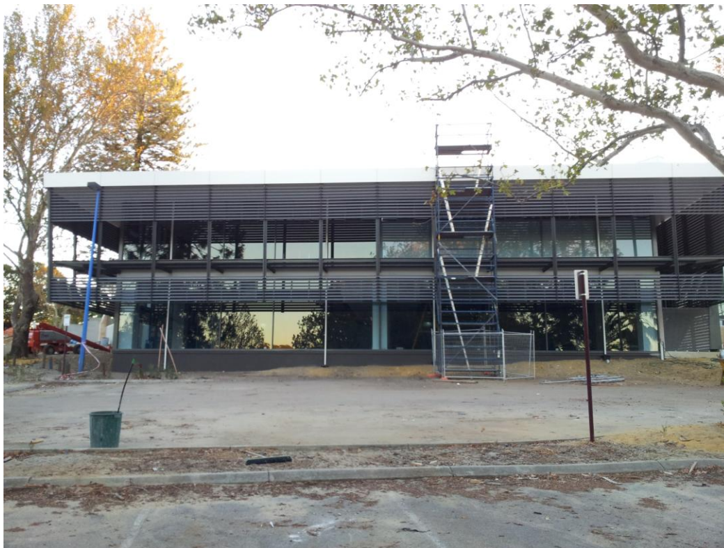
Ground Floor Aerobics Rooms and Top Floor Gymnasium
