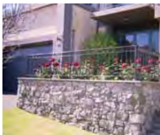
Open style fencing helps create a friendly neighbourhood and increases security through passive surveillance.
