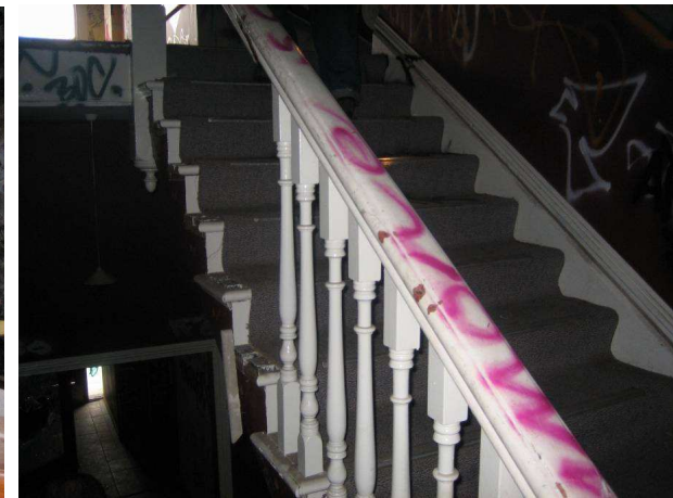
Balustrade of Central Stair
