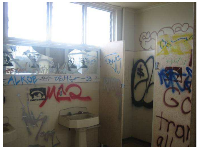
First Floor Toilets
