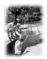
Facelift for Walcott Street: Engineering Services works crew lower a stormwater drainage manhole liner into position at the intersection of Walcott and William streets, Mt Lawley.
