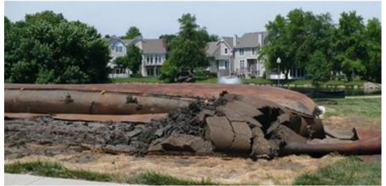
Envirotubes being cut open to enable the dry material to be removed.
