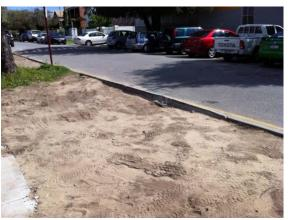
There is a trip hazard (and kerb damage) caused by vehicles continually parking on the verge.
