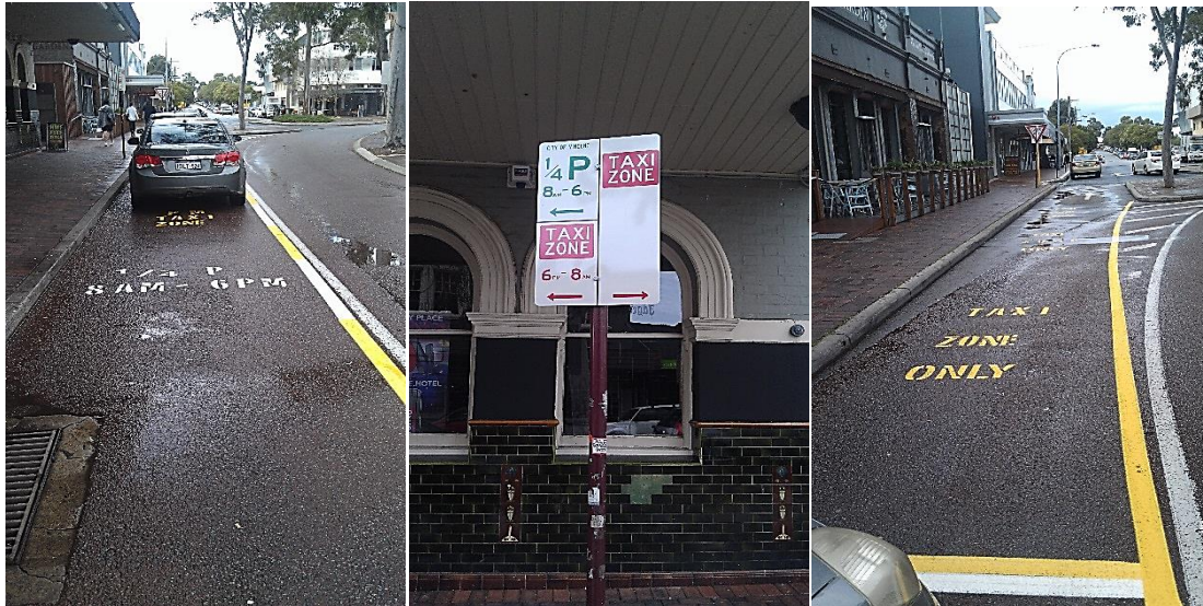
The split 1/4P and exclusive taxi zone as installed in 2013
