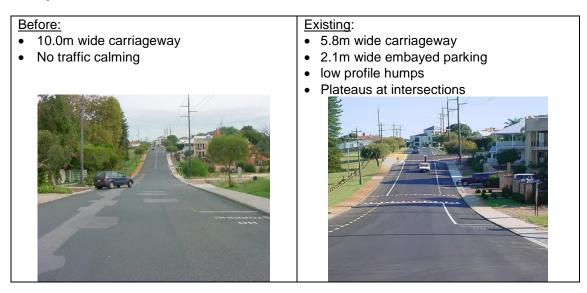
The traffic calming implemented at the time was designed to accommodate buses, as the street was on a bus route. With the removal of the bus route there is scope to implement additional measures to manage the speed and volume of traffic in the street.
