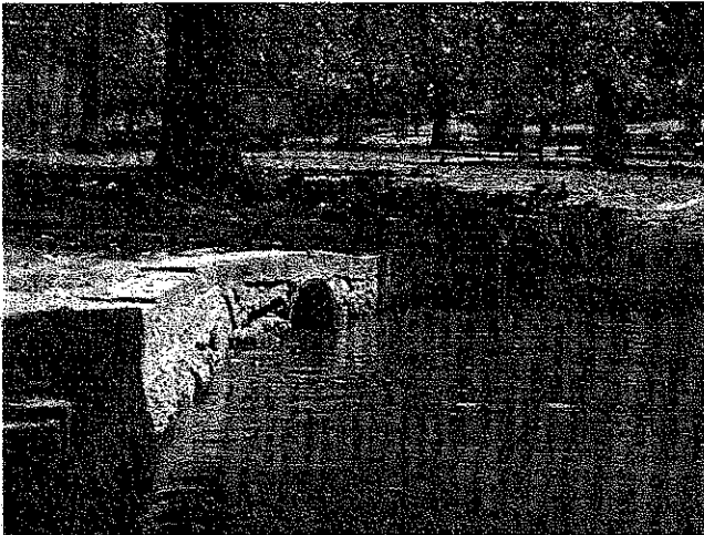
Record Photograph 48 Detail of retaining wall to the edge of lake. (April 2003)
