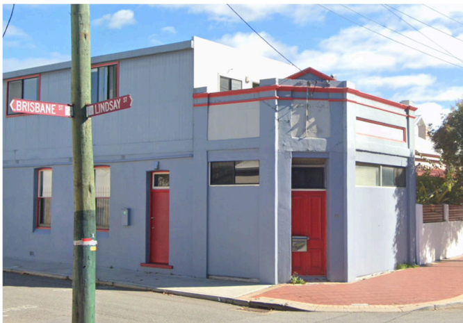
Figure 1: No. 99 Brisbane Street – View Looking West from Brisbane Street
