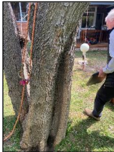
Image taken by Arbor Centre facing North – showing fluting at ground level
