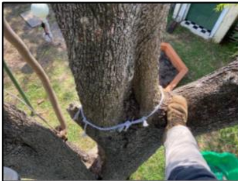
Image taken by Arbor Centre from within canopy – showing fluting within the canopy
