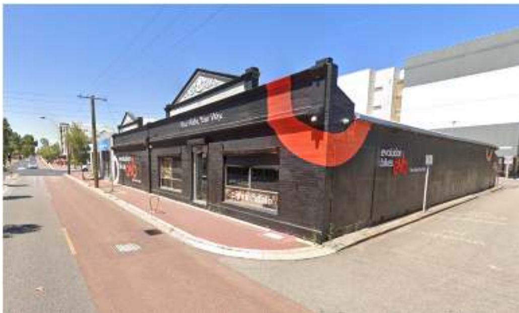
Figure 2 – Subject site during current operation in January 2023 with roller shutters open (Source: Google Street View)
