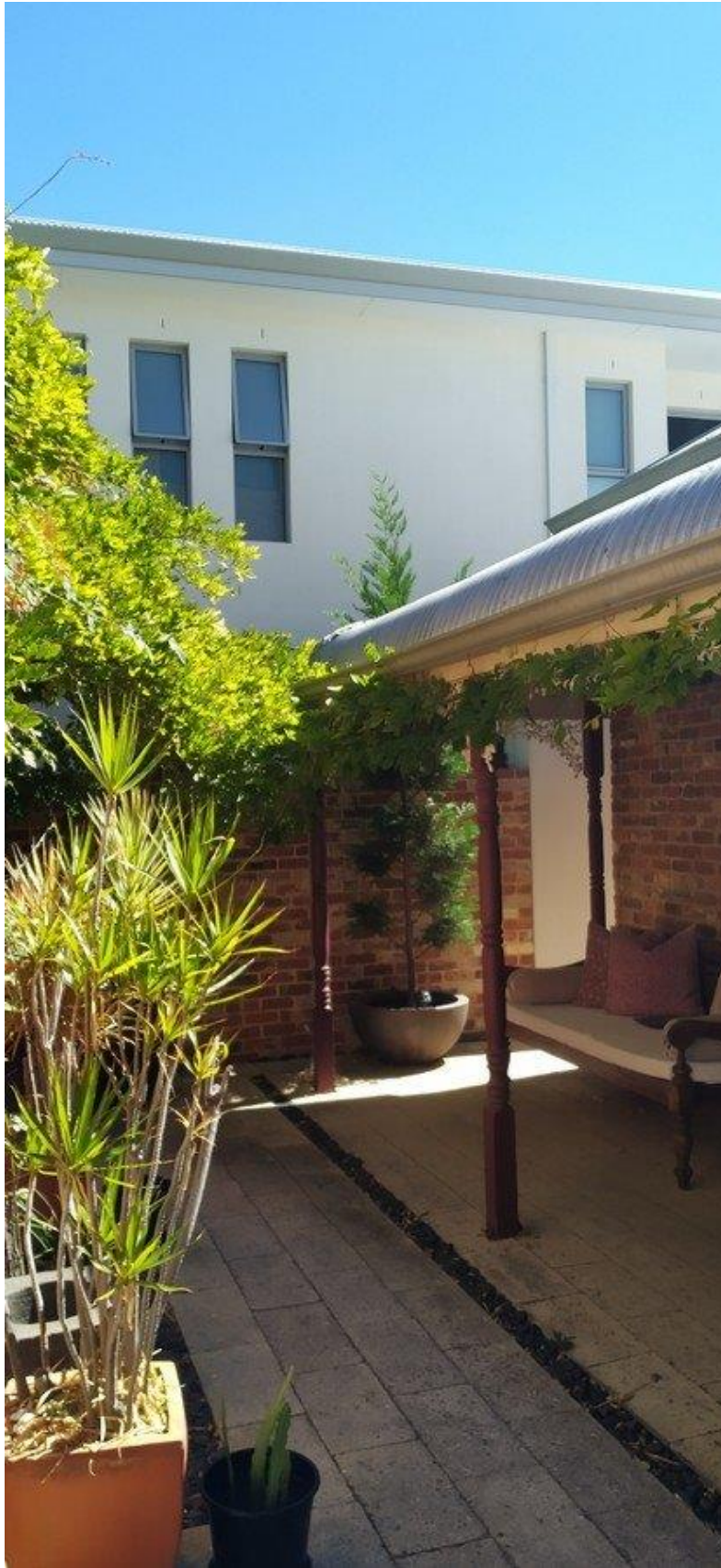
Figure 9: Existing two storey dwelling at 59 Glendower St provides a much more imposing wall with very little by way of articulation and appears to have a minimal setback to the western interface with 57 Glendower Street – this has a much greater bulk and scale impact in comparison to what is proposed to the opposite side.
