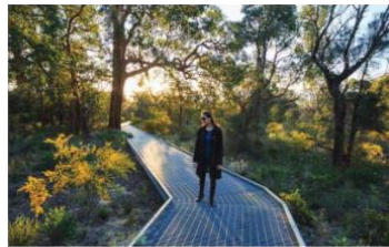
Figure 55. Raised perforated steel boardwalk.
