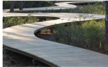
Figure 54. Example of raised timber boardwalk.
