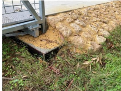
Plate 8 Path erosion protection
