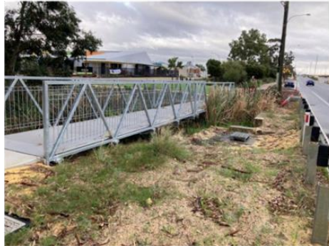
Plate Steel Truss bridge – City of Gosnells
