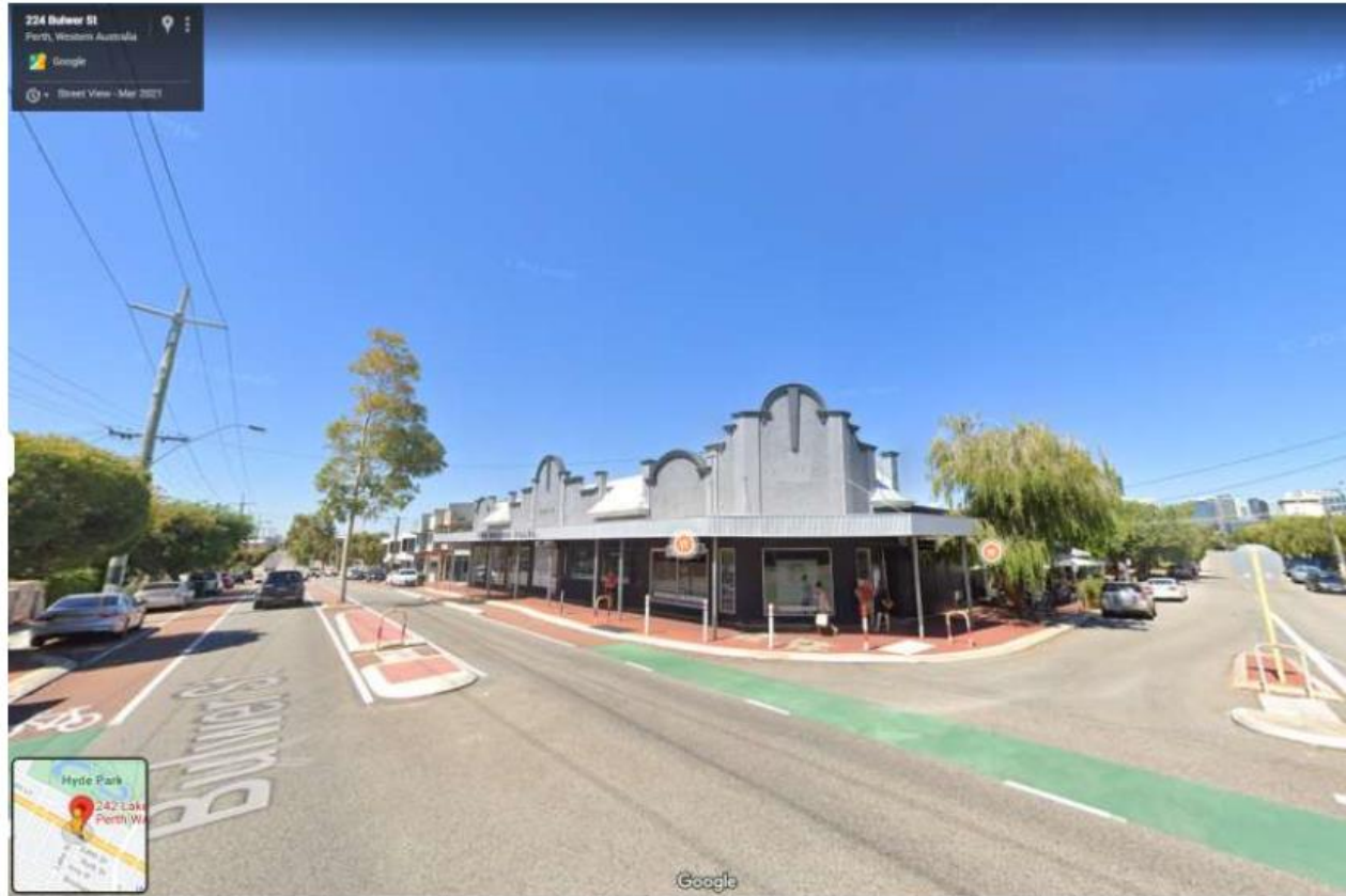
215-229 Bulwer Street – Traditional Single Storey Commercial Development
