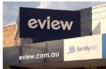
Above awning sign
