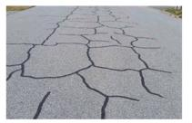
An interim crack sealing, - preventative n life of the asset (Fleet St – Access Road)
