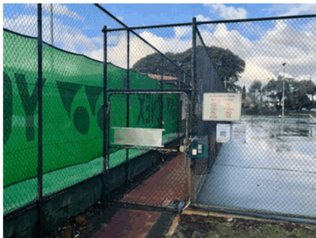
The existing entrance to the sports centre.
