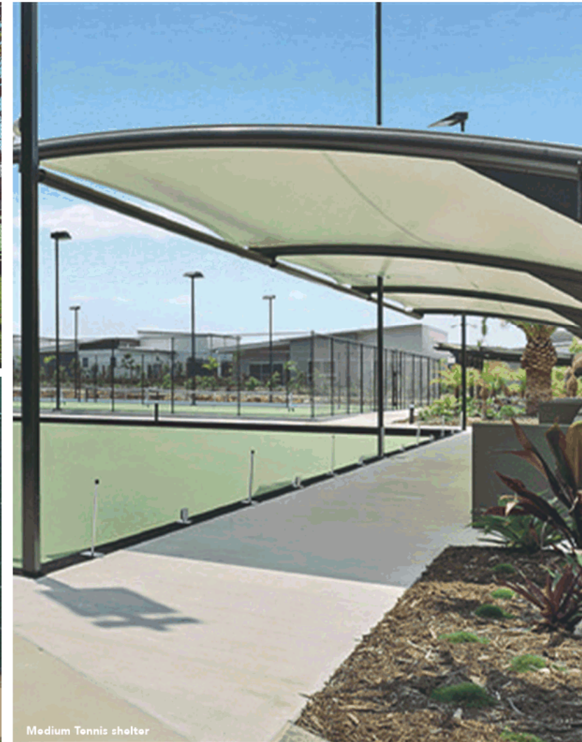
Medium Tennis shelter
