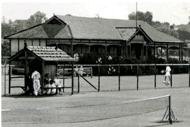
The original timber tennis pavilion and shelters of Robertson Park; 1930s.
