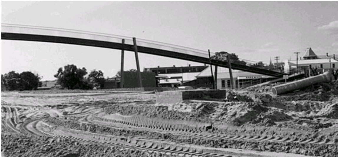
Construction of the Mitchell Freeway Leederville, 1974, COV PH00364
