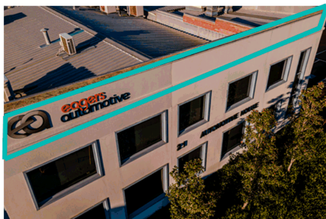
Roof signs are affixed parallel to the fascia but do not project above the roof line.
