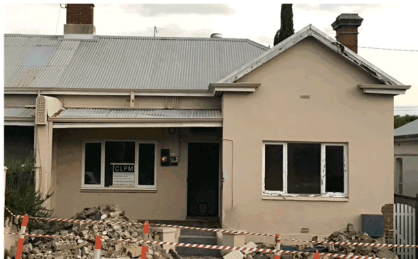
26 Moir Street Conservation Works (removal of obtrusive elements)
