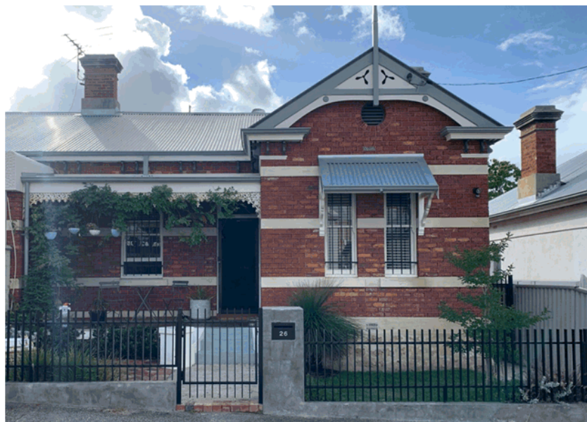
26 Moir Street Conservation Works (completion)
