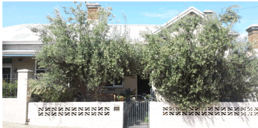
26 Moir Street Conservation Works (before)
