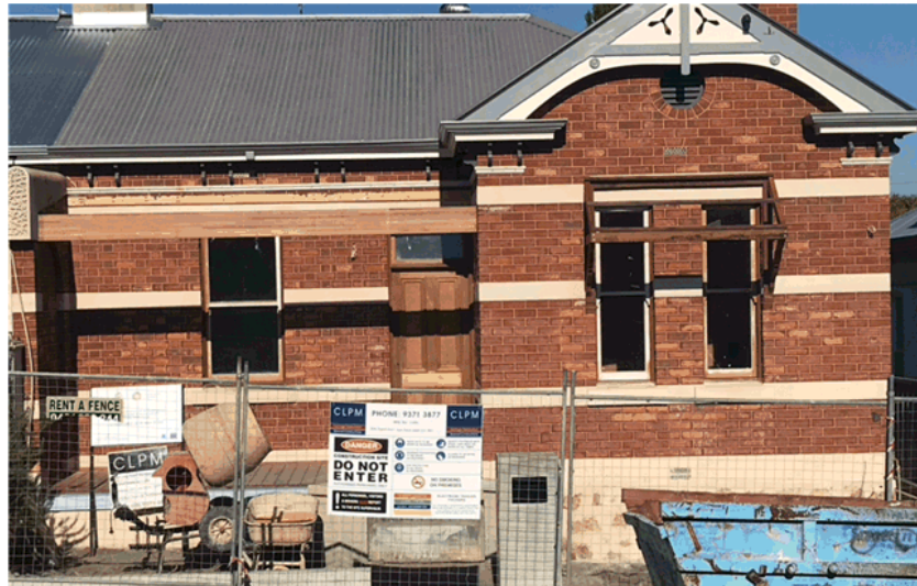
26 Moir Street Conservation Works (reinstatement of original features)
